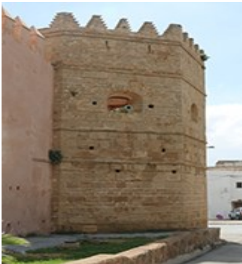
Fig. 9- the hexagonal tower
