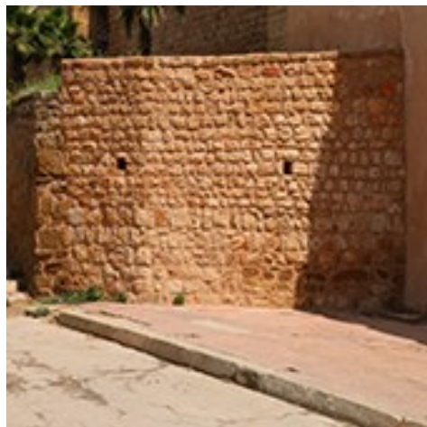
Fig. 2- Almoravid wall restored in late 2010
