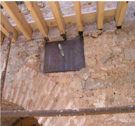
Fig.7- Consolidation of the vault
