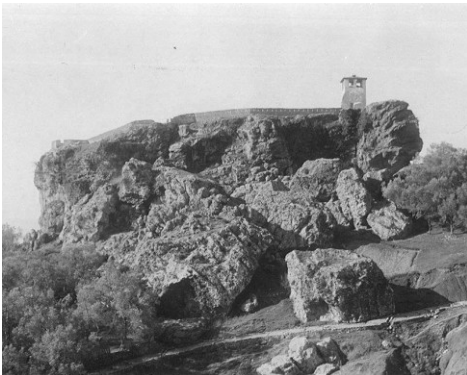
Fig. 2- South-eastern view of the castle
