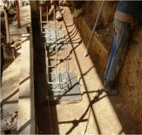
Fig. 6- Consolidation of the gallery
