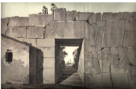
Fig. 2- Main gate of the fortress of Alatri (Dionigi, 1809)
