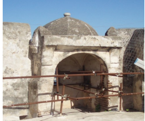
Fig. 4- View of the ribbed dome
