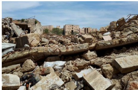
Fig. 9- Destruction around the citadel (SANA, 2016)
