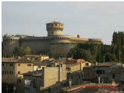
Fig. 3- Image of the “Mastio” of the Florentine Fortress of Volterra
