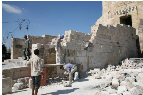
Fig. 10- Restoration of the citadel entrance (DGAM October, 2017) 5
