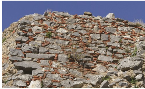
Fig. 12- Leontari- uncoursed rubble masonry with extensive use of ceramic fragments (2016)
