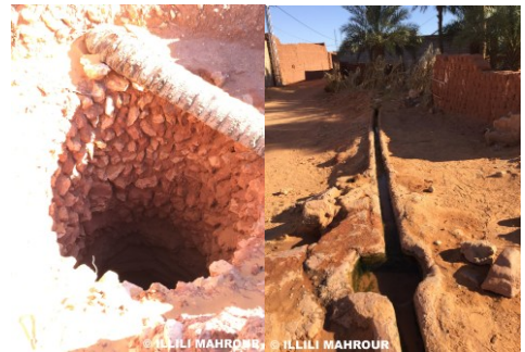
Fig. 5- Worked stone masonry well and Ifli in Agham Iffine gardens, Semjane. (Mahrou, 2018)
