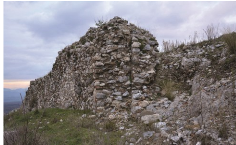
Fig. 6- Leontari. Early Ottoman reinforcement of defensive wall's width (2016)
