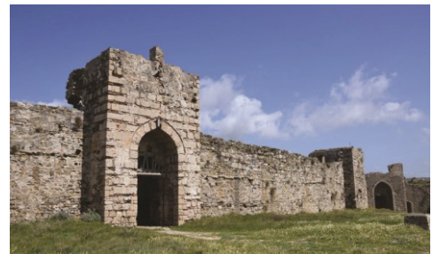
Fig. 11- Modone- Typical Ottoman construction on the diving wall (2018)
