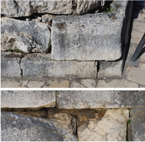
Fig. 11- Regular-shaped blocks (up) at the corners of the bastion, and the remains of cramps and lead (down), bastion Priuli (author)
