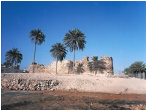
Fig. 5- Keshm Fort with constructive elements added above the parapet (Campos, 2002)
