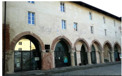
Fig. 3- Casale Monferrato castle today; portico in the first courtyard
