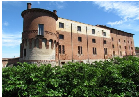
Fig. 1- Saluzzo Castle, view overlooking the hillside
