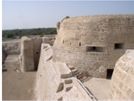
Fig. 10- The round bastion of the great South curtain and an orillon casemated bulwark at the corner of the ditch (Campos, 2005)
