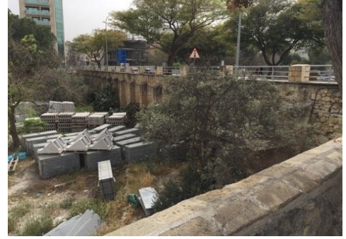
Fig. 1- Passage between Costanza-D'avila Bastion (by Author, 2018)
