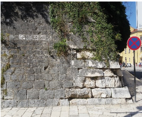
Fig. 12- Regular-shaped blocks at the corners of the bastion, and carved stone blocks of slightly smaller dimensions for the rest of bastion scarpa , bastion Priuli (author)
