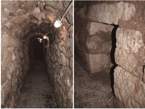
Fig. 7- Contramine gallery (on the left) and the entrance to the small room (right), eastern demibastion (author)
