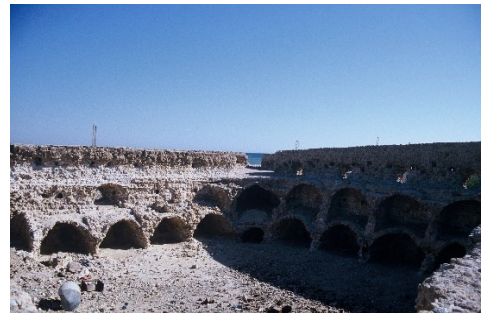
Fig. 6-7- (Campos, 2004) - Larak Fort, view from outside and inside, with posterior addition of constructive elements over the vaulted platform of terreplein of the fortification
